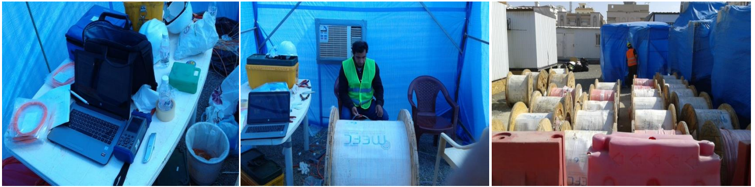
Fiber Optic Cable Drum Test (SECo Jeddah)
