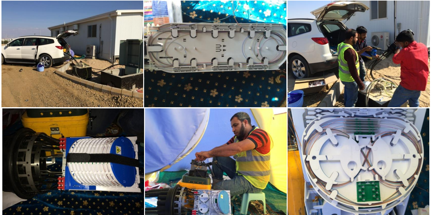
Fiber Optic Splicing at STC Site ARAMCO RABIQ
