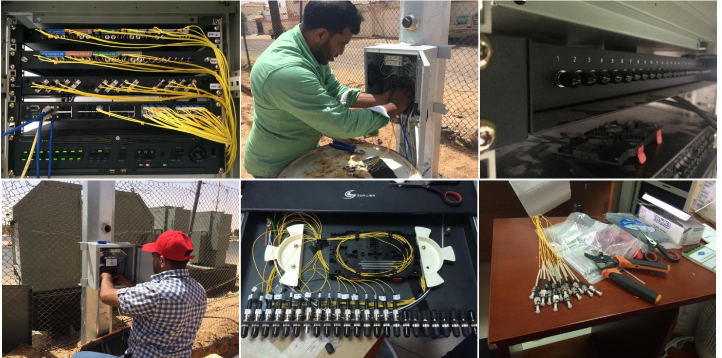
Fiber Optic Splicing for IP Camera (SECo Sharurah)
